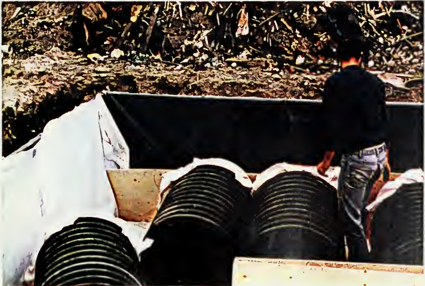
A9: INSTALLATION OF BIG "O" STORAGE ZONE TILE.
